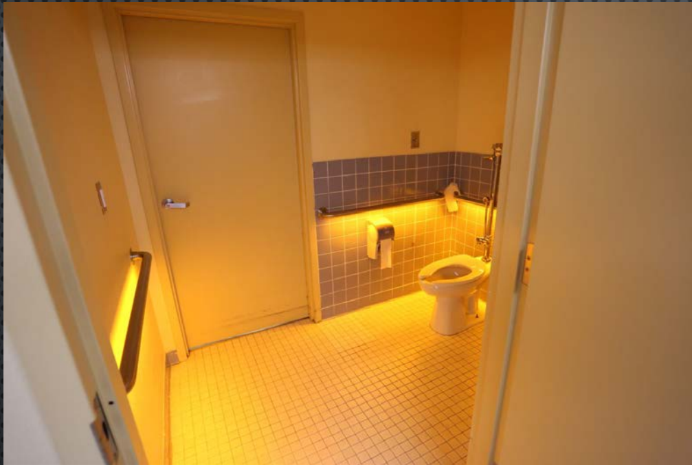
Bathroom lighting Photo: Connie Samla ACC Care Facility
